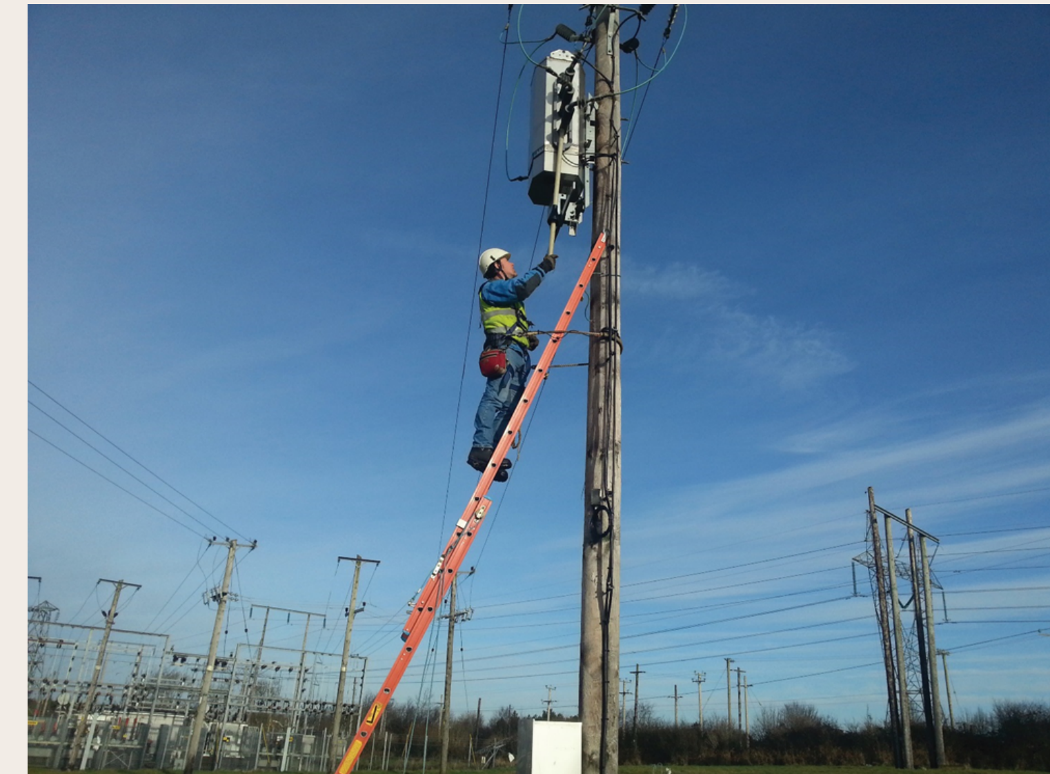
Installing new devices at one of the ESB trial sites in Ireland
